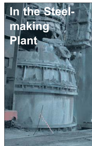
Converter 3 is of prime importance to SMS for the realization of the steelmaking production schedule.
